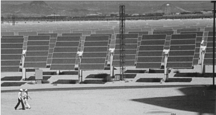
Figure 6-3. Solar mirrors at the Solar One Power Plant. Each mirror stand has a surface area of 39 square meters. Showing the two men reveals how large the mirrors are.
